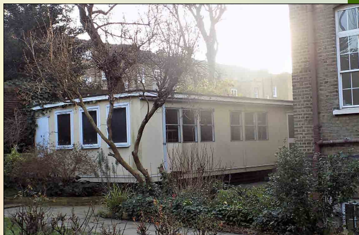
The 30 year old portakabin classrooms
